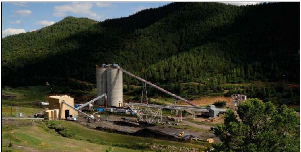
Image: Aerial view of the Mine: ROM and Product pads; CHPP; and twin storage silos.
